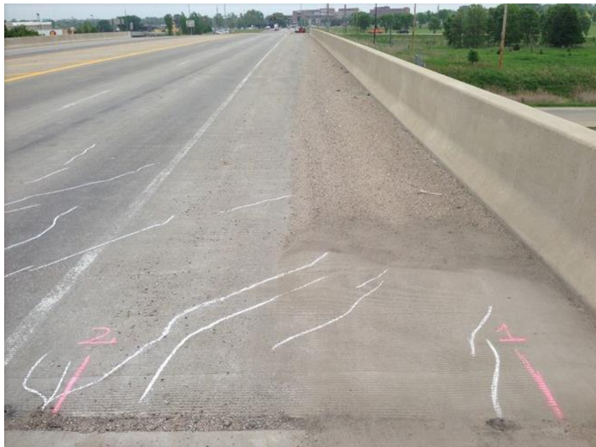
Figure 5. Longitudinal cracks at middle of deck top
