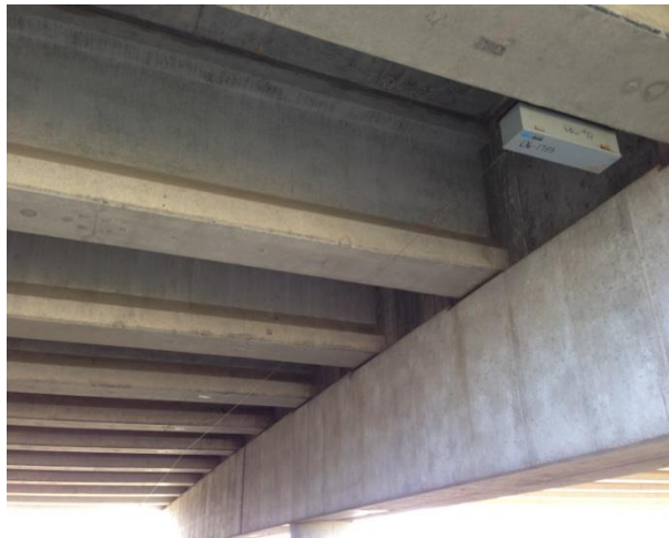
Figure 18. Vibrating wire long-range displacement meter
